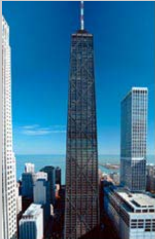
John Hancock Building
